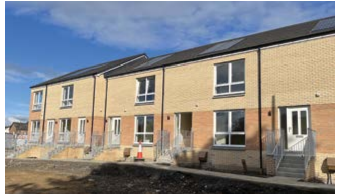
Johnston Avenue (Phase 2), Cornton – nearing completion
