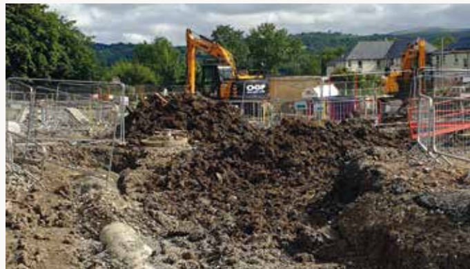
Under construction, Drip Road, Stirling.
