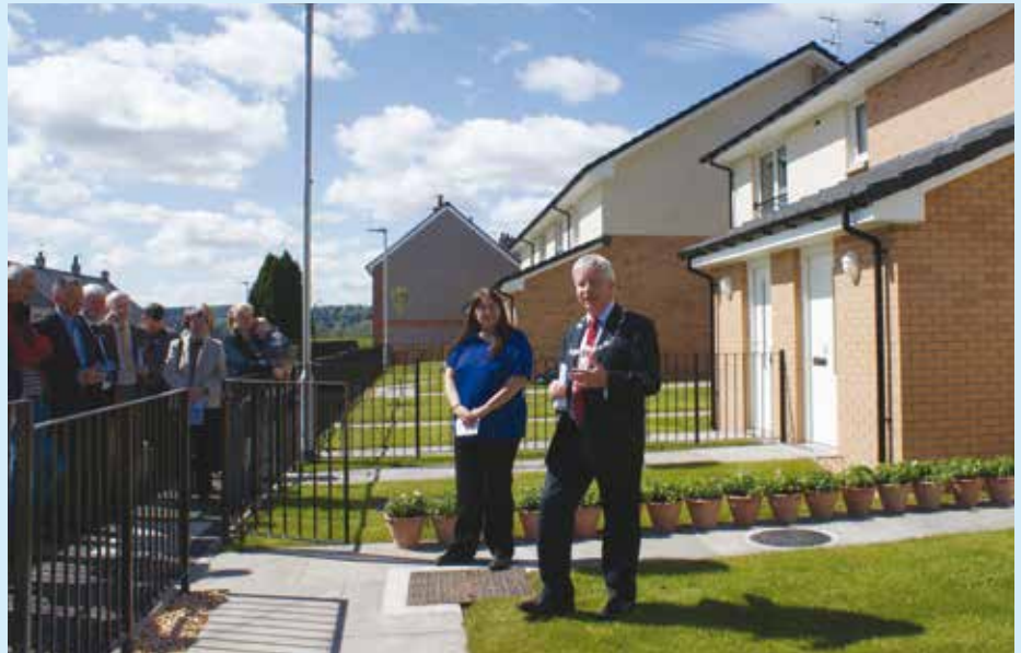
Provost Robbins and Forth's Chairperson mark the completion of Cultenhove Crescent
